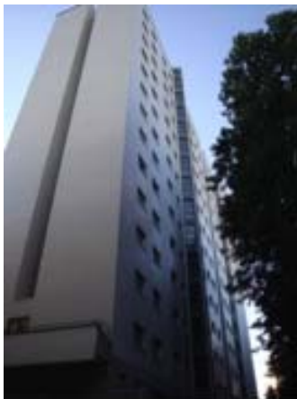
IMAGE 6: Façade with Mosaic tiles and repeated openings. Service corridor along the height of the building
